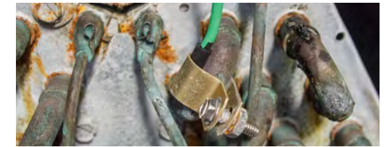
Installing temperature sensor of the QwikSwap™ on the coil
